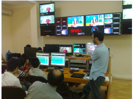
Police TV - Master Control Room
