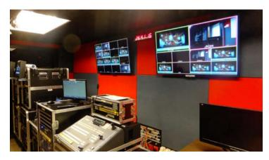
The playout of broadcast playlists is performed by a redundant Etere Automation system, which along with Etere MTX and Xor-Media servers gives a truly multi-format playout that doesn't require media conversions. Etere MTX is the best of breed IT solution for media servers, it provides fast access to video contents while providing Logos and Crawls overlaying and traditional Master Control capabilities.
